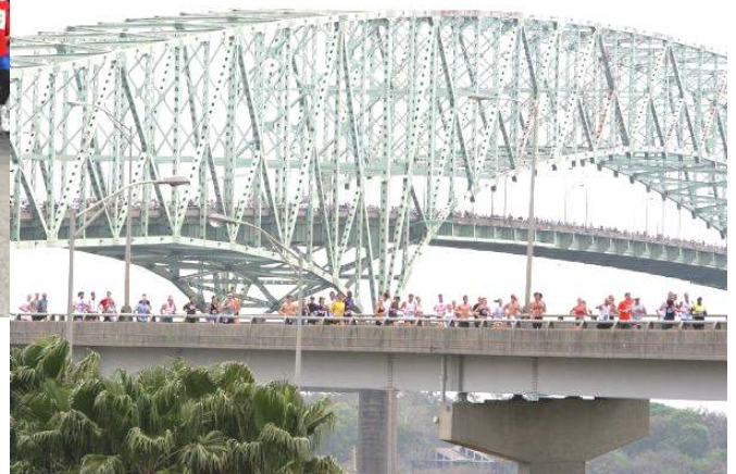
2006 GATE RIVER 15K HART BRIDGE
